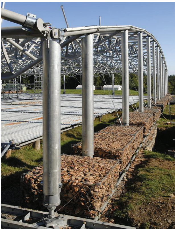
Fig. 3. Type 1 of a support structure – non-invasive structure from the Bibracte site in France (designed by P. Andreu, Tess Atelier D'Ingénierie; source: https://www.tess.fr/en/projet/excavation-shelter )
