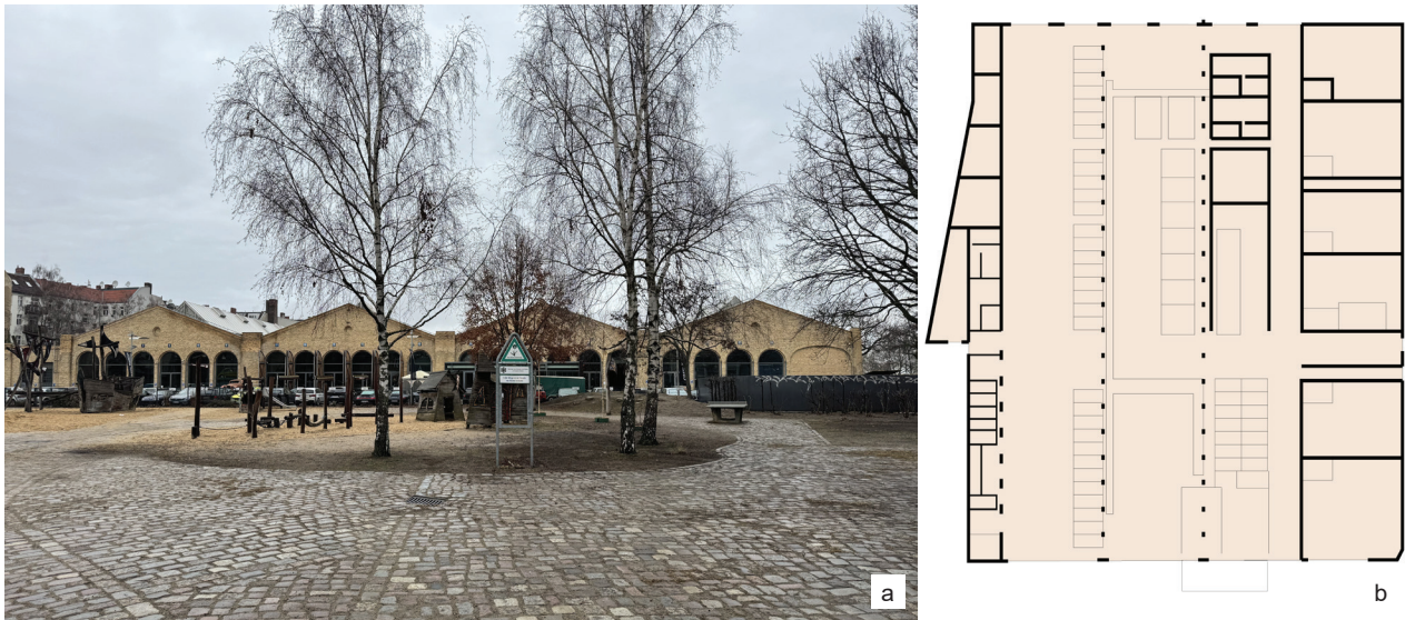
Fig. 5. Tram depot on Wiebestraße in Berlin, embedded within a city block and transformed into the multifunctional automotive centre Classic Remise: a) front façade from the interior of the block, Wiebestraße (photo by A. Czajczyńska-Mieszala), b) building plan (elaborated by A. Czajczyńska-Mieszala)
