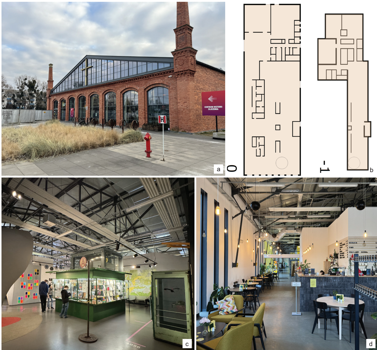
Fig. 6. Former tram depot in Grabiszyńska Street in Wrocław, located outside the compact urban fabric and adapted into the Depot History Centre: a) front façade from Grabiszyńska Street, b) building plan, c) exhibition area inside the museum, d) entrance and gastronomic zone (photos and elaborated by A. Czajczyńska-Mieszala)
