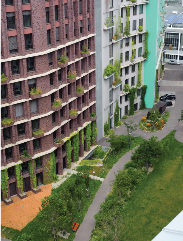
Fig. 8. Green façades made of vines in the Biotope City development in Vienna (photo by A. Gierko, 2022)
