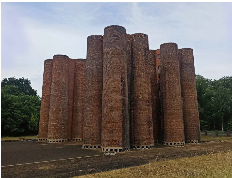
Fig. 4. Biotürme, old coke production furnaces in Lauchhammer, revalorized as a part of IBA Fürst-Pückler-Land (photo by P. Sołowiej, 2023)
