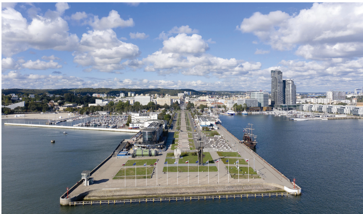
Fig. 10. The South Pier – the main architectural feature of the city (source: Heritage Protection Department of Gdynia City Council, photo by B. Ponikiewski, 2022)
