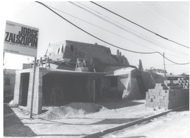
Fig. 6. Construction of Zalszupin's residence in Guarujá (20.07.1971) (source: © Acervo Casa Zalszupin)
